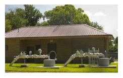
Baton Rouge Water Company currently operates a scavenger well system in the "1,500-foot" sand on North Street between N. 31<sup>st</sup> and N. 32<sup>nd</sup> streets to protect the at the Lula Street Pumping Station from further saltwater encroachment. Nearly four years of data show the "scavenger" system to be working as predicted.
